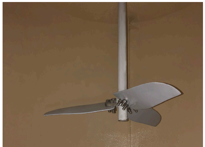
4. Finished interior of mixing tank with restored mixing blades.
